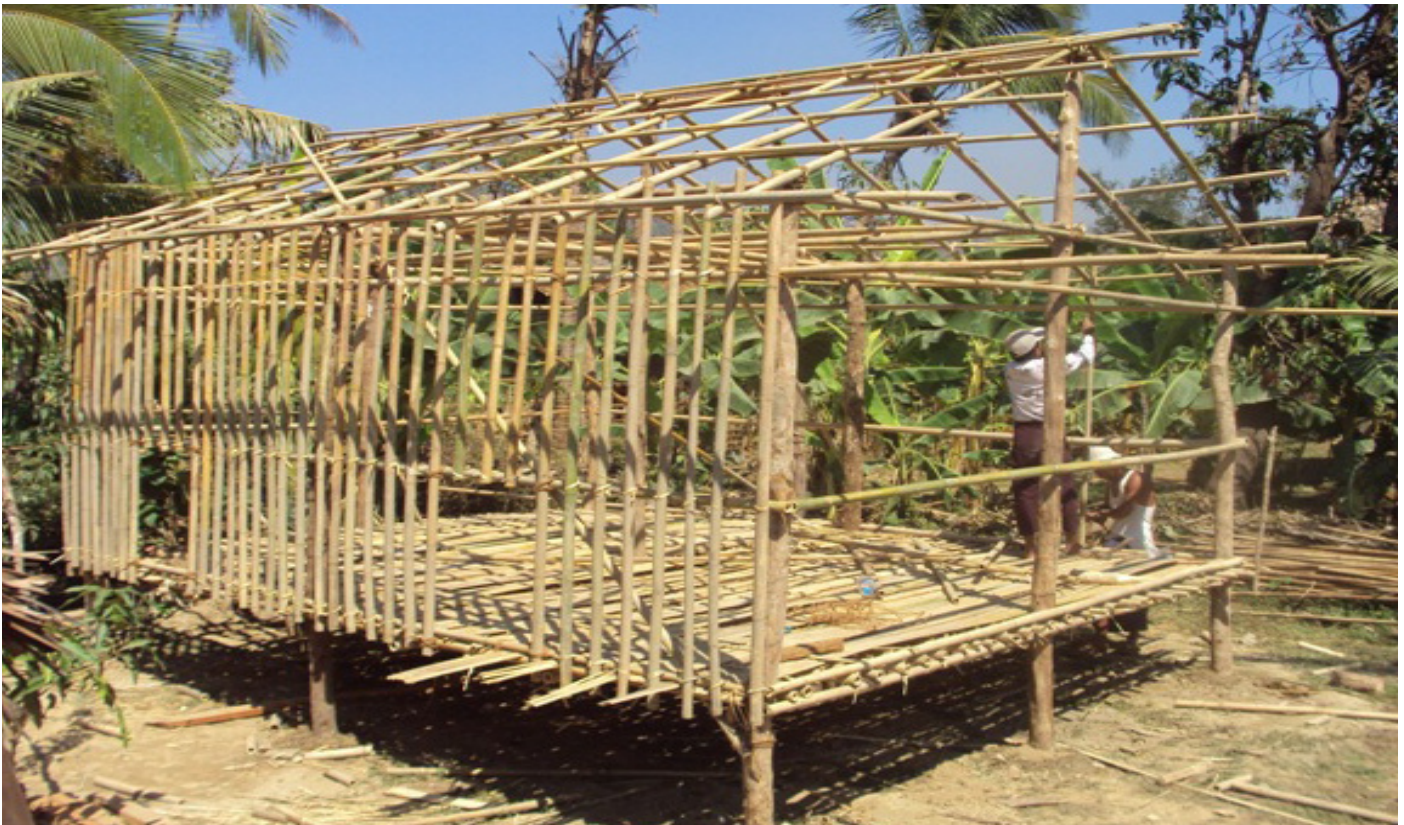
Shelter under construction at Oak Kan village
