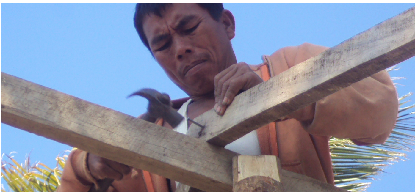
Construction of model houses
