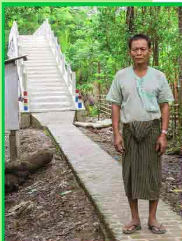
CARE capped its continuous five-year Nargis response efforts for Hla Than's Aye Su village with a bridge to access health and education services.
