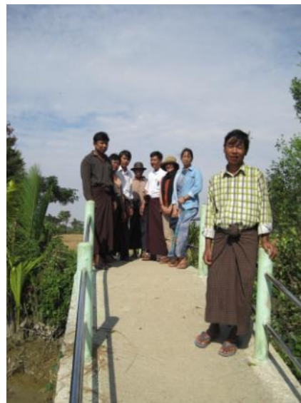
Bridge constructed in village in Wa Thay
