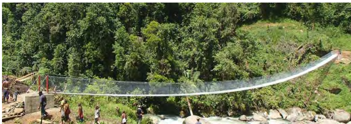
Figure 10 - Completed swing iron footbridge near Simbari with a span of 76m
